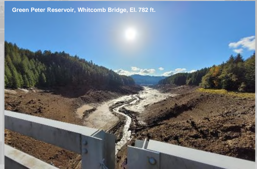
Green Peter Reservoir, at El. 782 ft.
