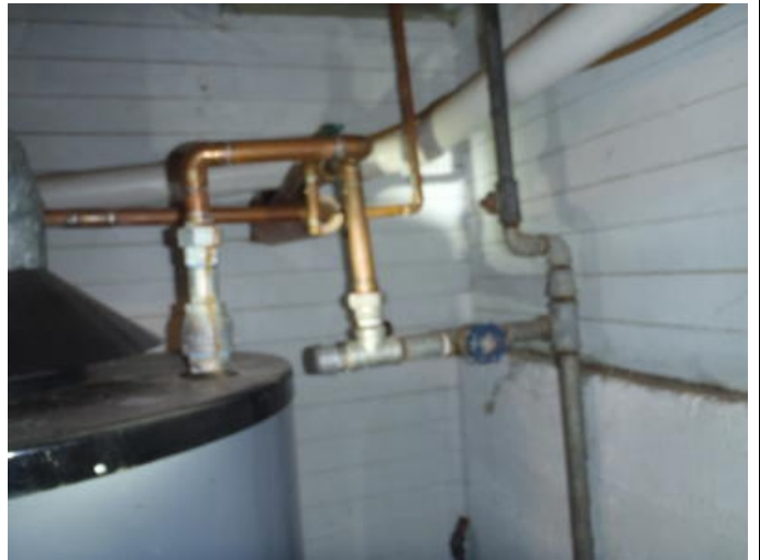
Photo #548 Water & Waste Pipe – Galvanized /Copper &
