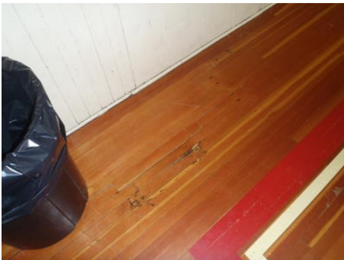
Photo #413 Floor Cover - Gym – Wood
