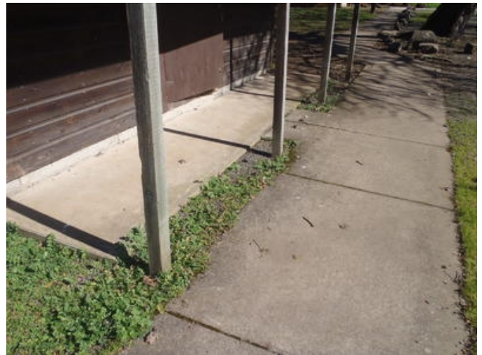
Photo #178 Landing – Concrete
