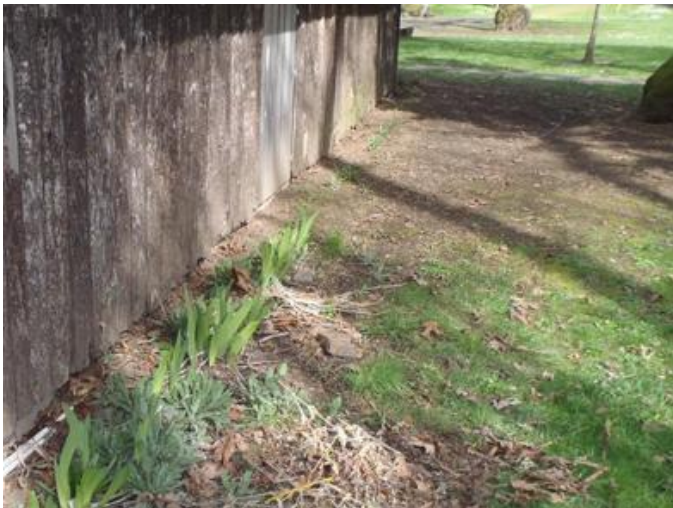
Photo #296 Landing – Concrete
