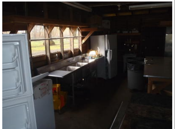
Photo #282 Lighting - Bathrooms /Kitchen /Security /Art
