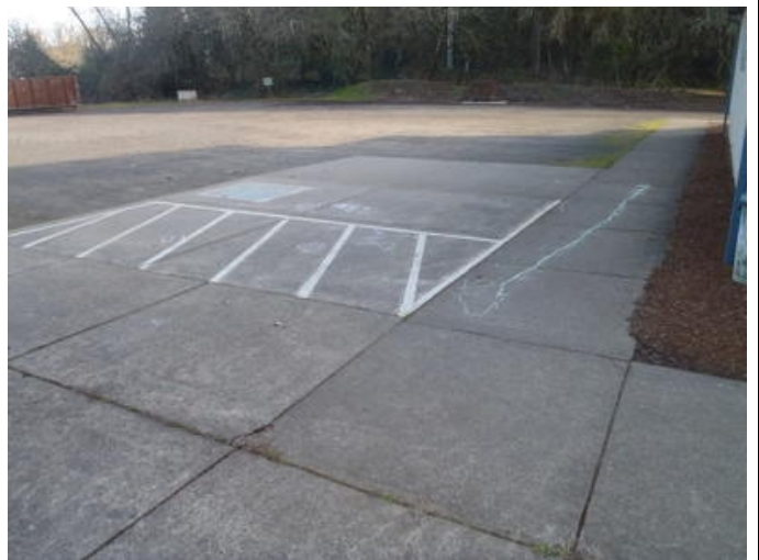
Photo #402 Curbing/Wheel Stop – Rocks & None
