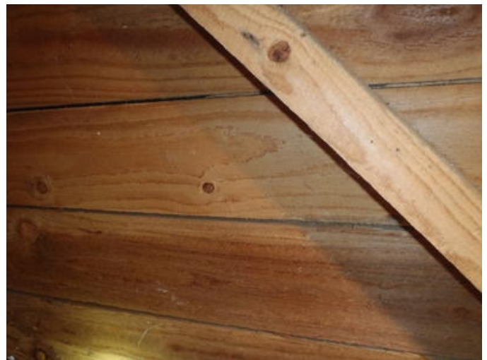
Photo #316 Substructure – Wood Studs only
