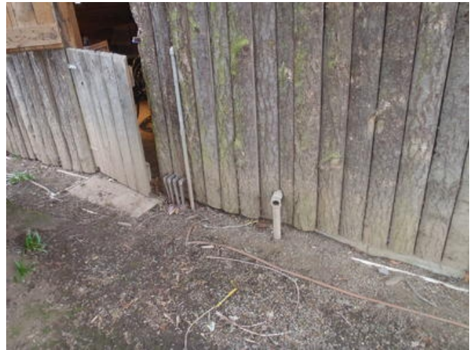
Photo #304 Landing – Concrete
