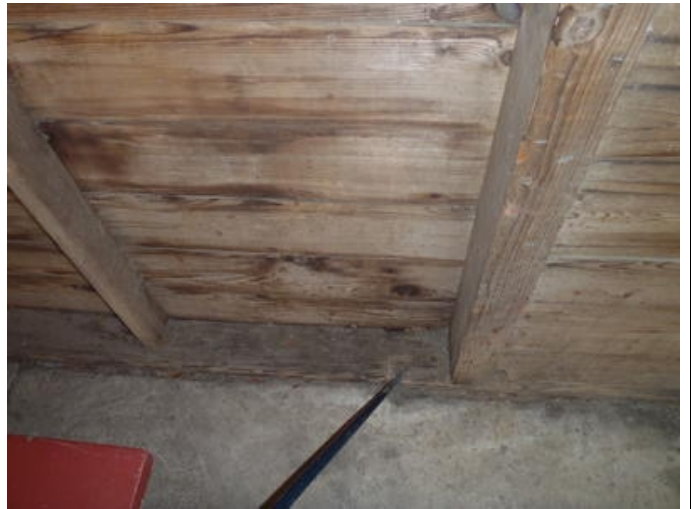
Photo #257 Substructure – Wood Studs
