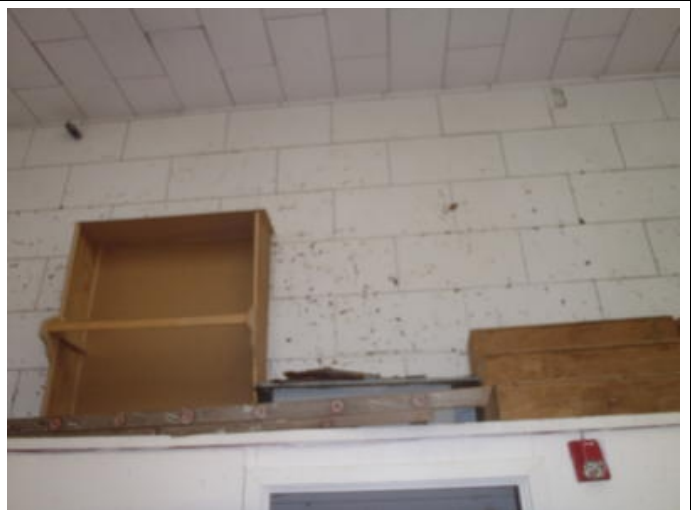
Photo #477 Ceiling & Wall – Paint
