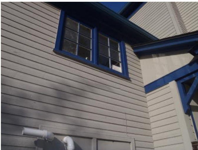
Photo #372 Window, Frames and trim. – Wood
