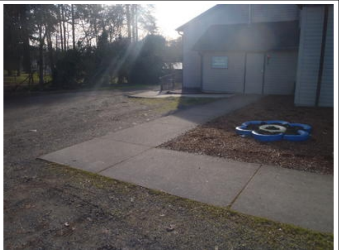
Photo #403 Walkways – Concrete
