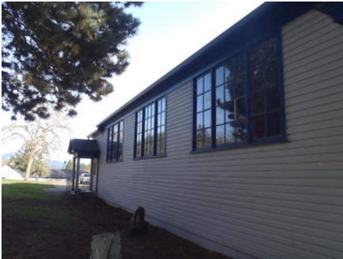
Photo #357 Window, Frames and trim. – Wood
