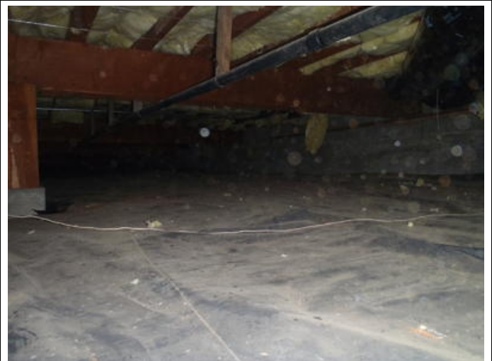
Photo #588 Insulation & Vapor Barrier – Fiberglass 6+\" &
