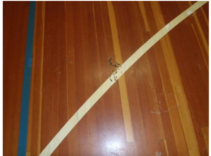
Photo #412 Floor Cover - Gym – Wood
