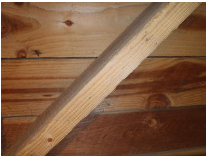
Photo #315 Substructure – Wood Studs only
