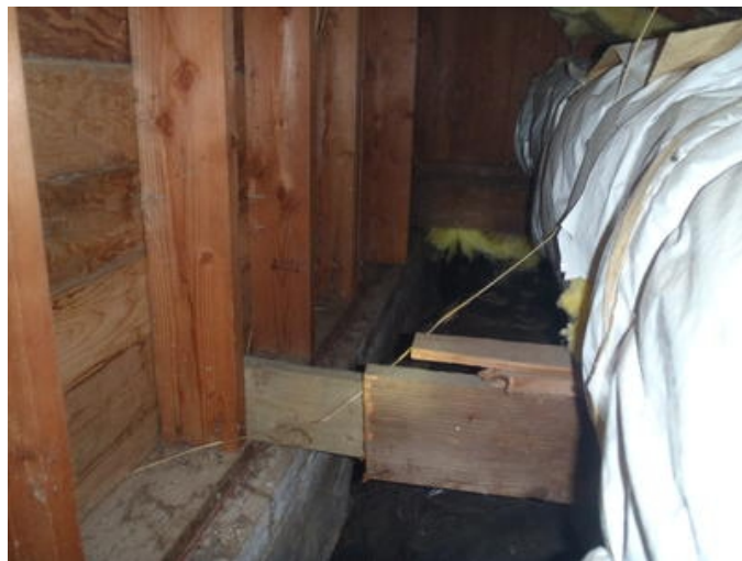
Photo #600 Wood Structure – Joist & Beam
