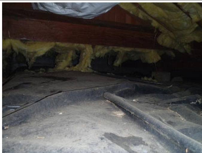
Photo #603 Insulation & Vapor Barrier – Fiberglass 6+\" &
