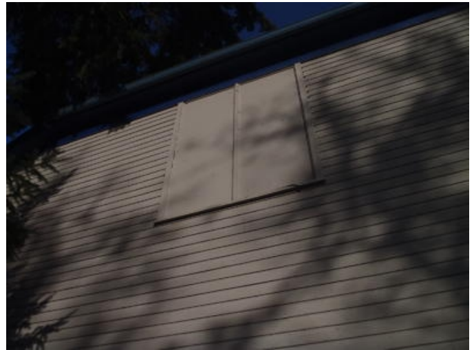
Photo #362 Window, Frames and trim. – Wood
