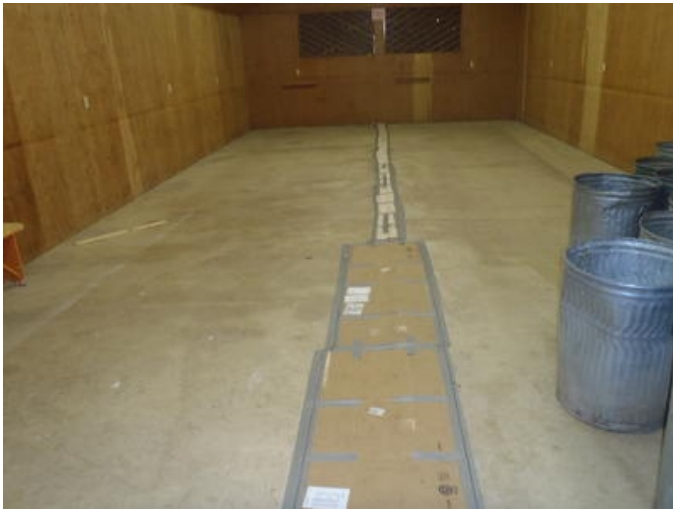
Photo #181 Foundation & Slab – Concrete
