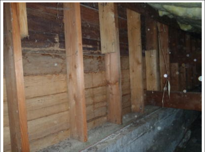
Photo #596 Wood Structure – Joist & Beam
