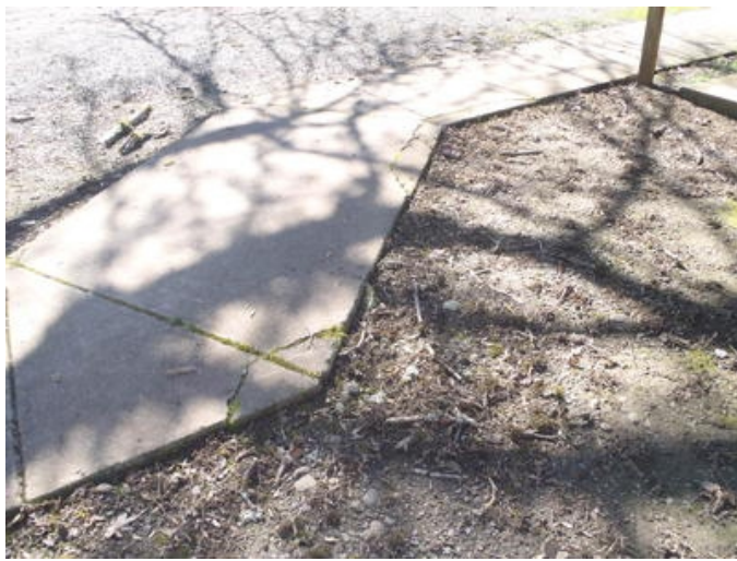
Photo #170 Walkways – Concrete
