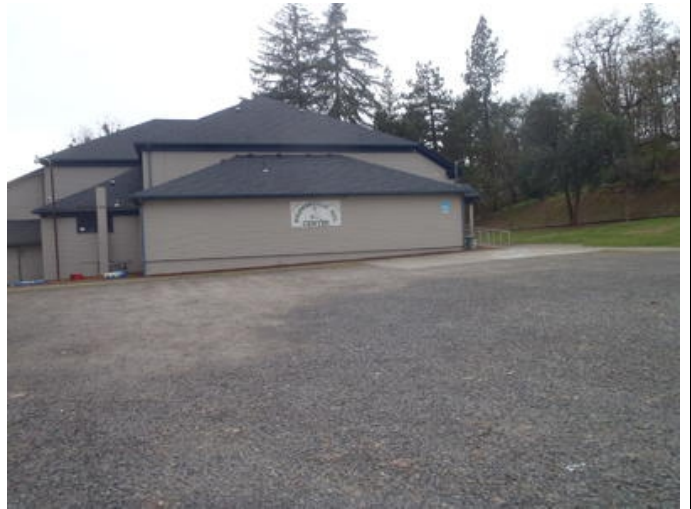
Photo #621 Parking & Road – Gravel
