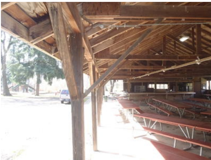
Photo #267 Substructure – Wood Studs
