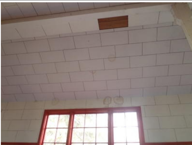
Photo #425 Ceiling & Wall – Paint
