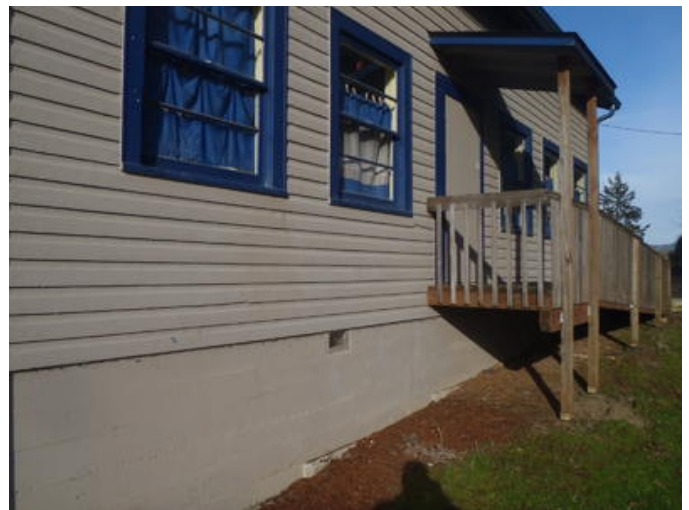
Photo #379 Window, Frames and trim. – Wood
