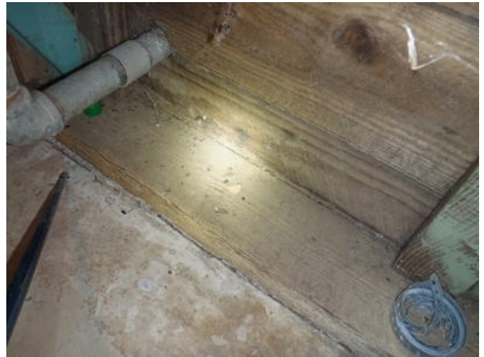
Photo #312 Substructure – Wood Studs only
