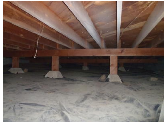
Photo #584 Wood Structure – Joist & Beam
