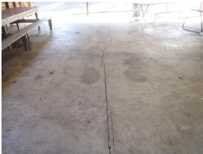
Photo #256 Slab – Concrete
