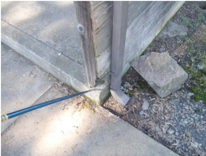
Photo #193 Substructure – Wood Studs
