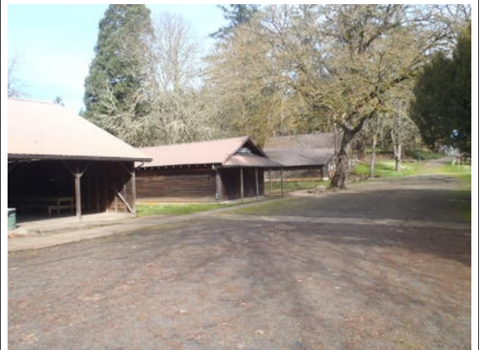
Photo #324 Site - Art Building –
