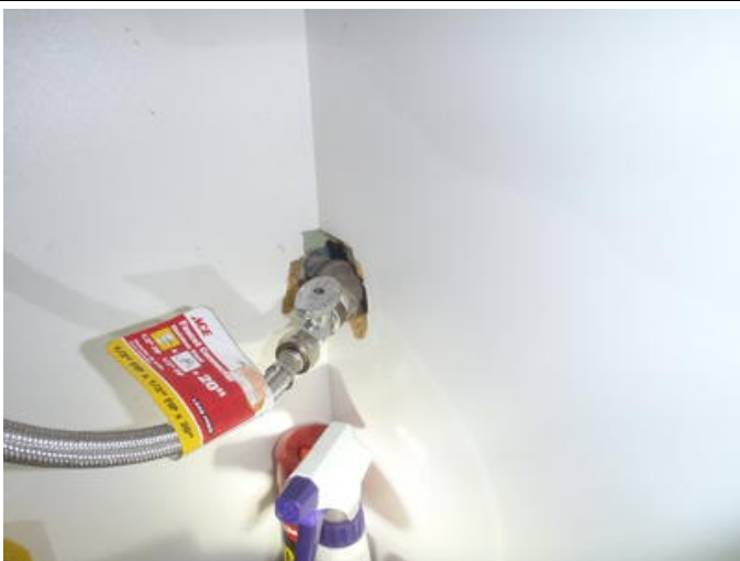
Photo #551 Water & Waste Pipe – Galvanized /Copper &
