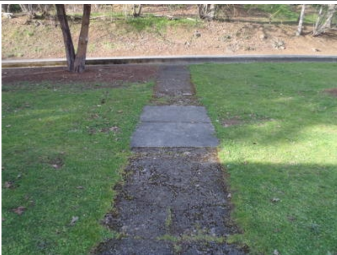
Photo #347 Walkways – Concrete
