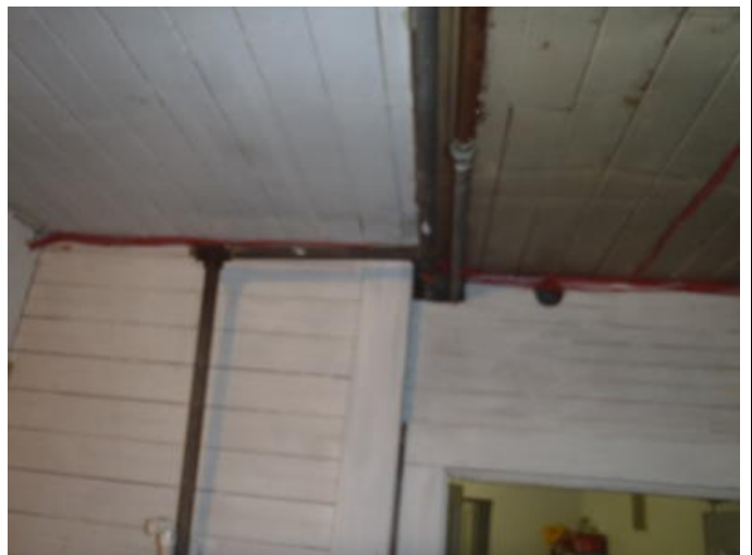
Photo #550 Water & Waste Pipe – Galvanized /Copper &
