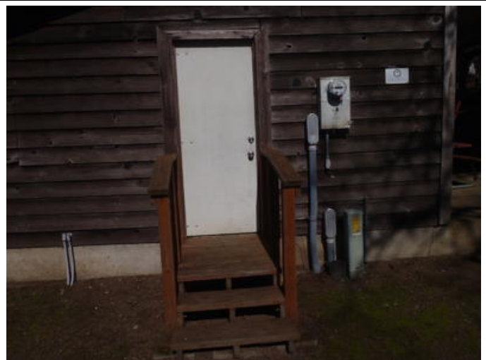
Photo #139 Stairway, Guardrail & Handrails – Wood
