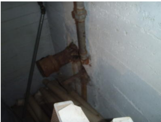
Photo #549 Water & Waste Pipe – Galvanized /Copper &
