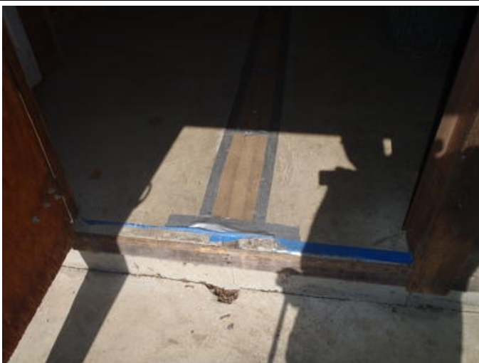
Photo #180 Landing – Concrete
