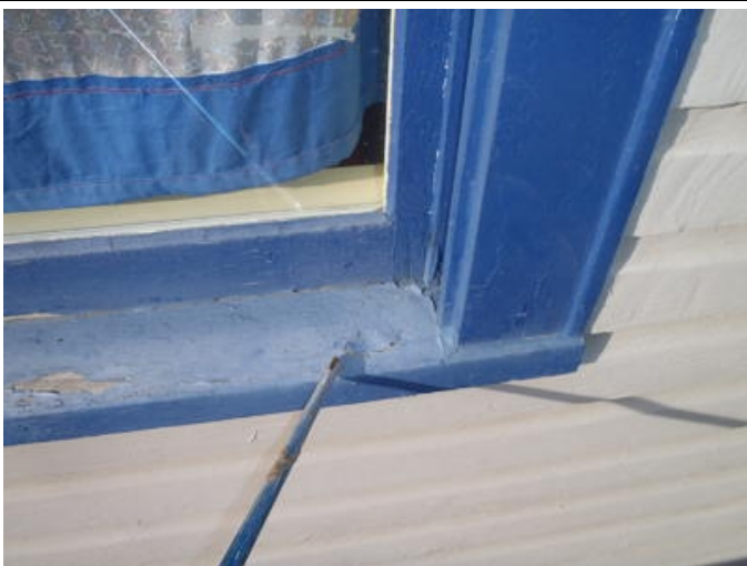
Photo #385 Window, Frames and trim. – Wood
