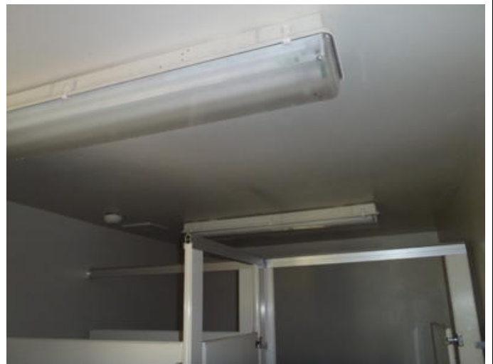
Photo #234 Lighting - Bathrooms /Kitchen /Security /Art
